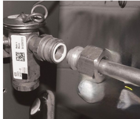
Figure 25. Seal placement
