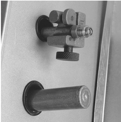
Figure 29. Schrader valve
