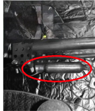
Figure 30. Sensing bulb
