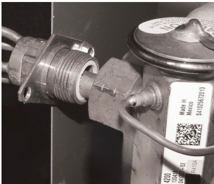
Figure 24. Swivel nut installation
