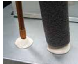
Figure 31. Seal the openings
