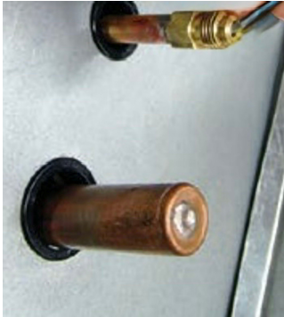
Figure 28. Nitrogen holding charge
