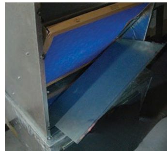
Figure 9. Bottom return application
